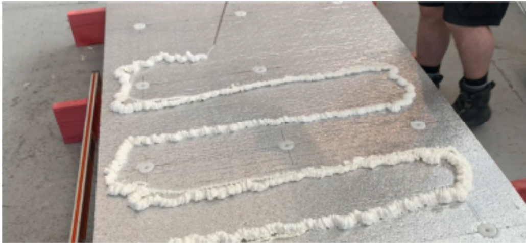
Figure 9-7. Applying Viking Soudafoam
